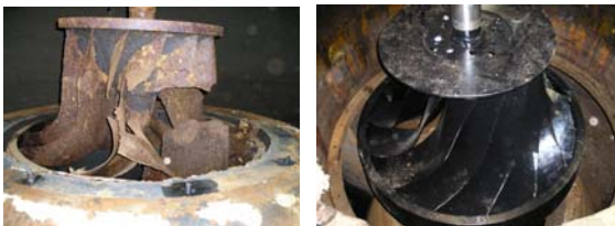
Removed and replacement hydro turbine
